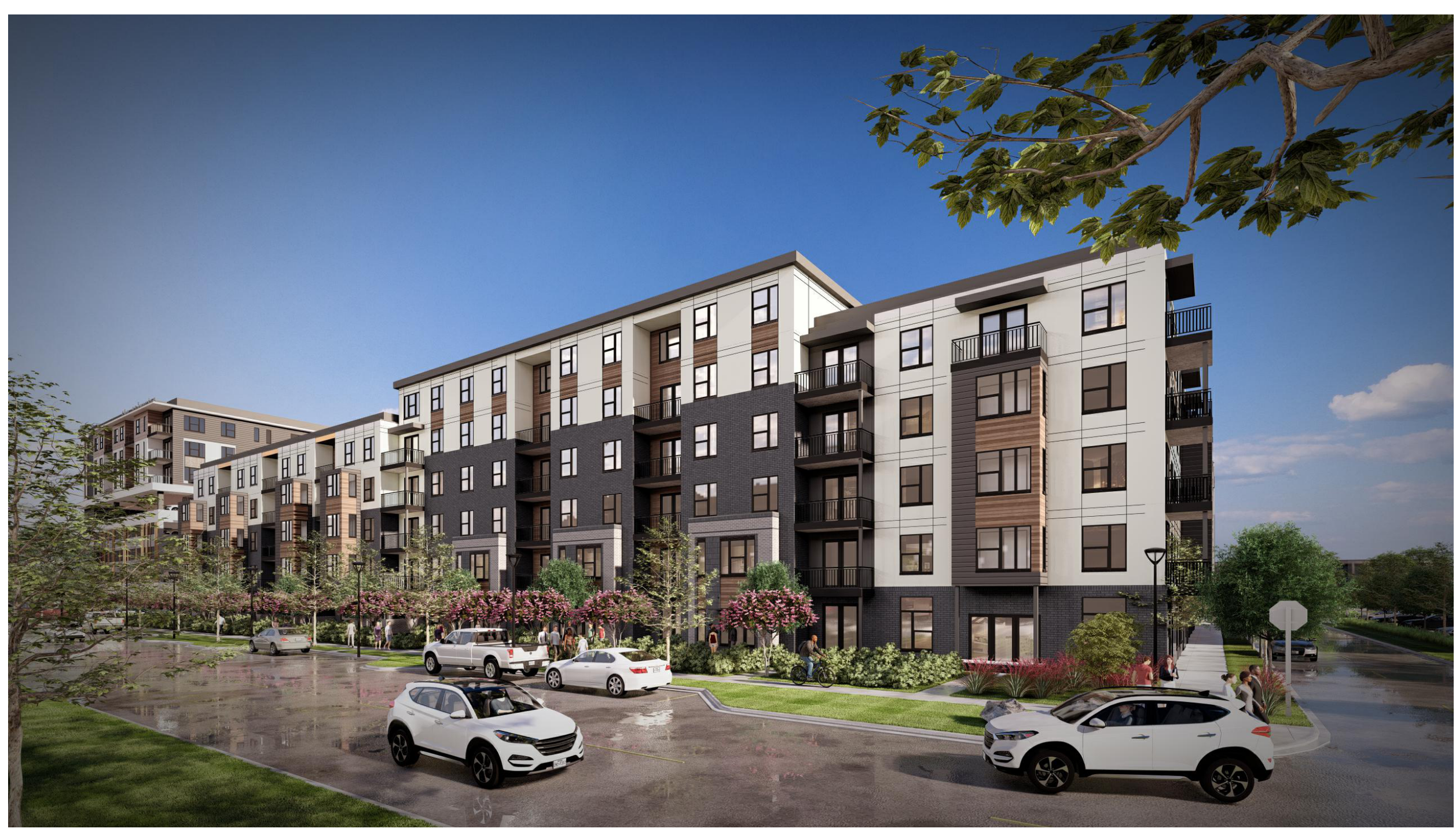
VIEW OF SOUTH FACADE AT LANDMARK BOULEVARD
