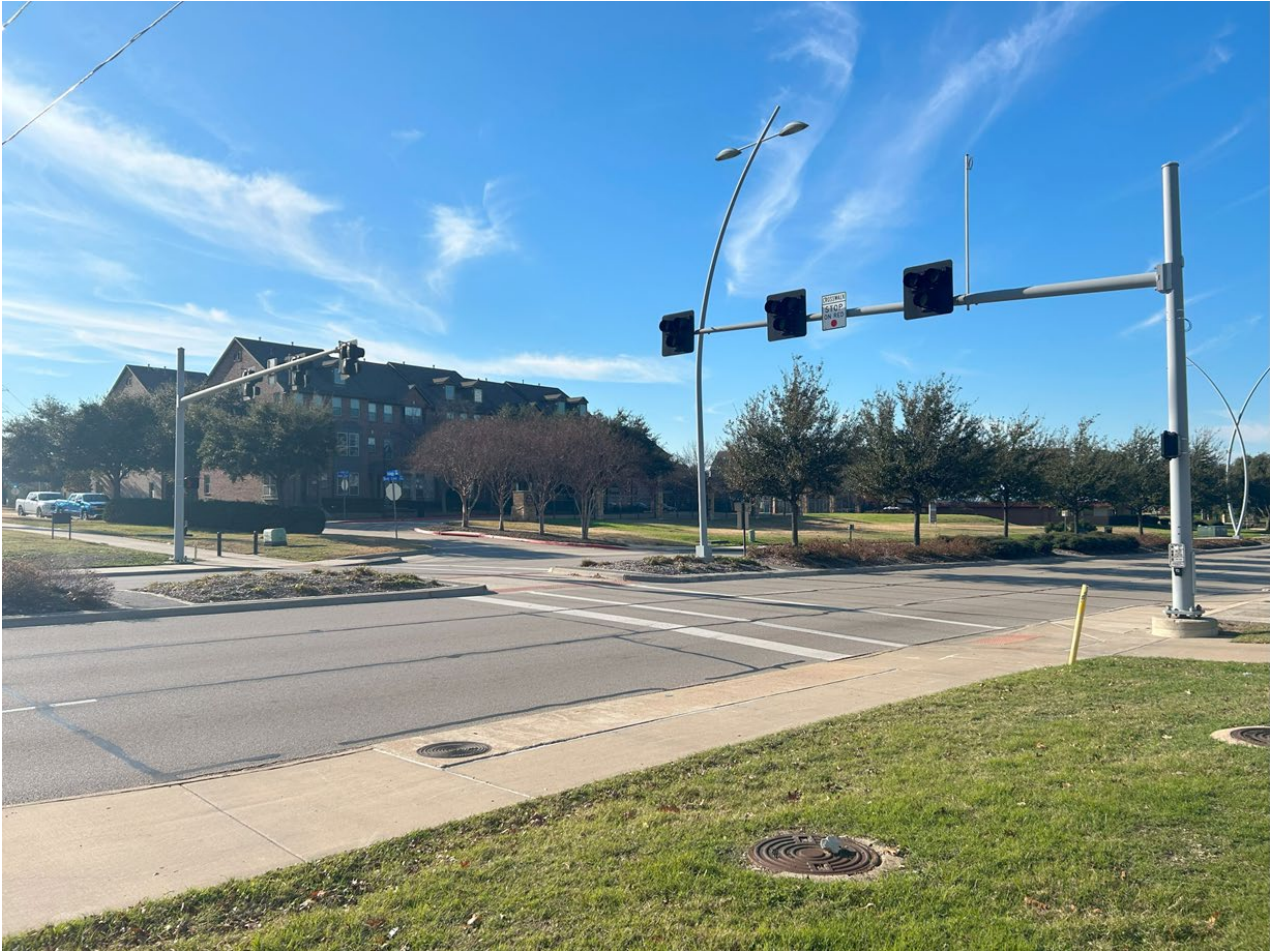
At Belt Line Road and Redding Trail
