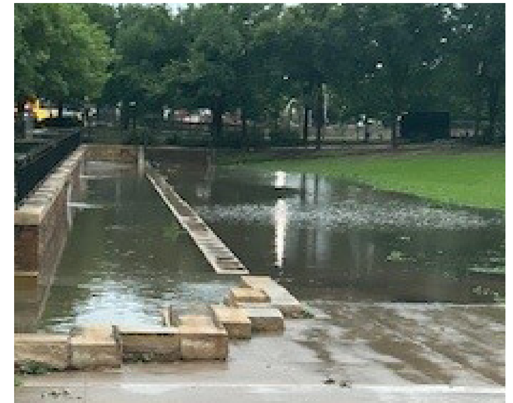
Grading and Drainage
