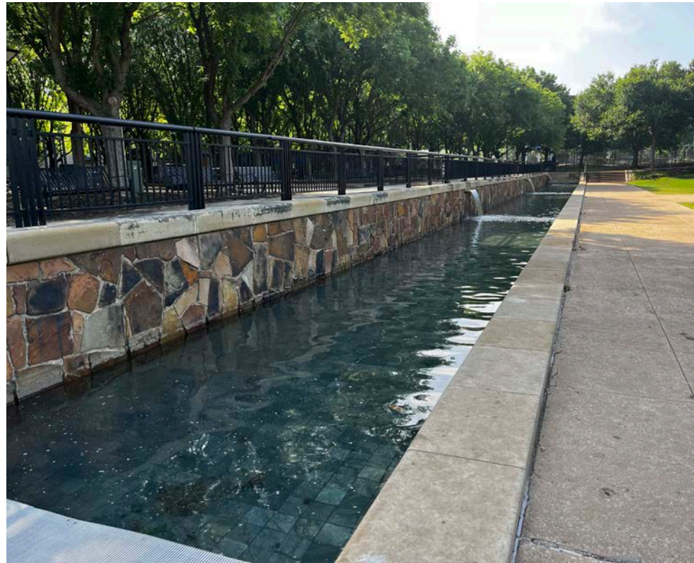
On-Going Water Feature Maintenance
