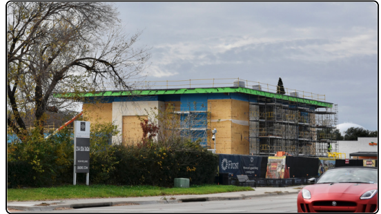
Frost Bank Under Construction
