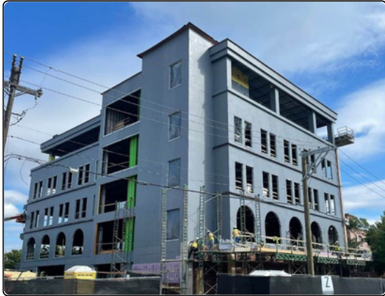
One Addison Place Under Construction
