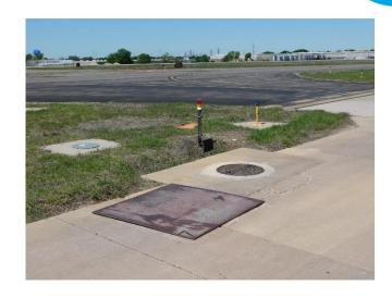
The vehicle service road has completely failed in multiple locations. A full-depth reconstruction is required. The reconstructed road will be two lanes wide (the current road is a single lane with traffic in both directions).
