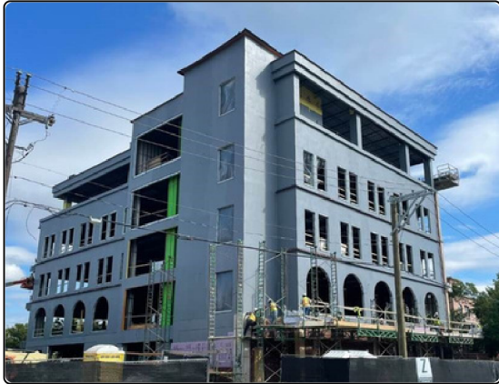
One Addison Place Under Construction
