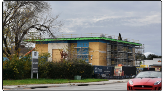
Frost Bank Under Construction
