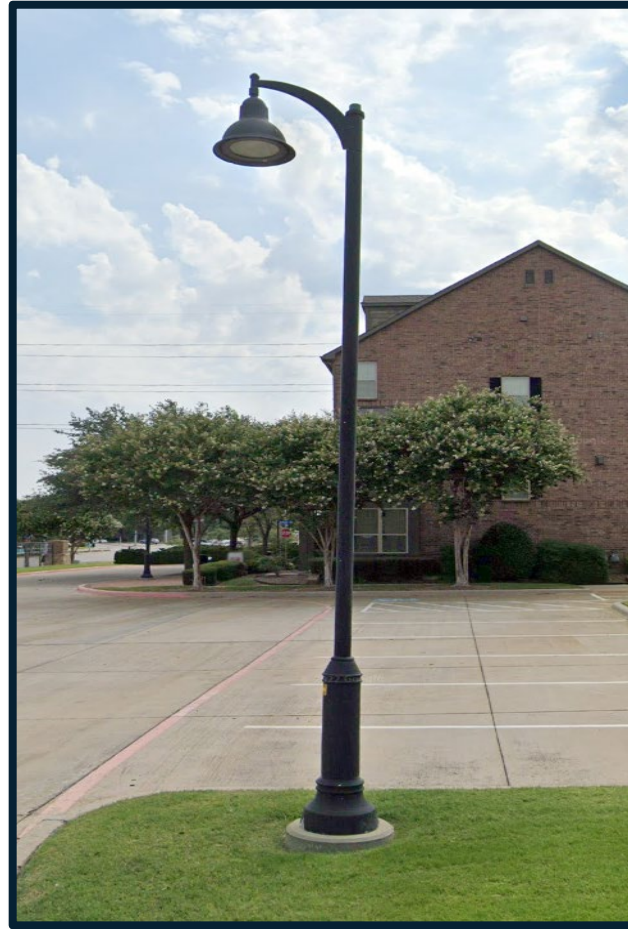
Decorative Light Pole Foundation
