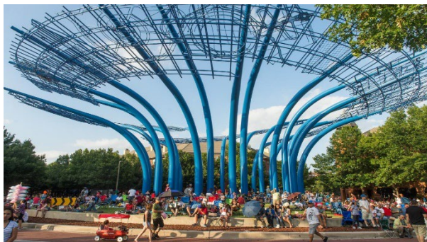
Addison Circle Park, Town of Addison
