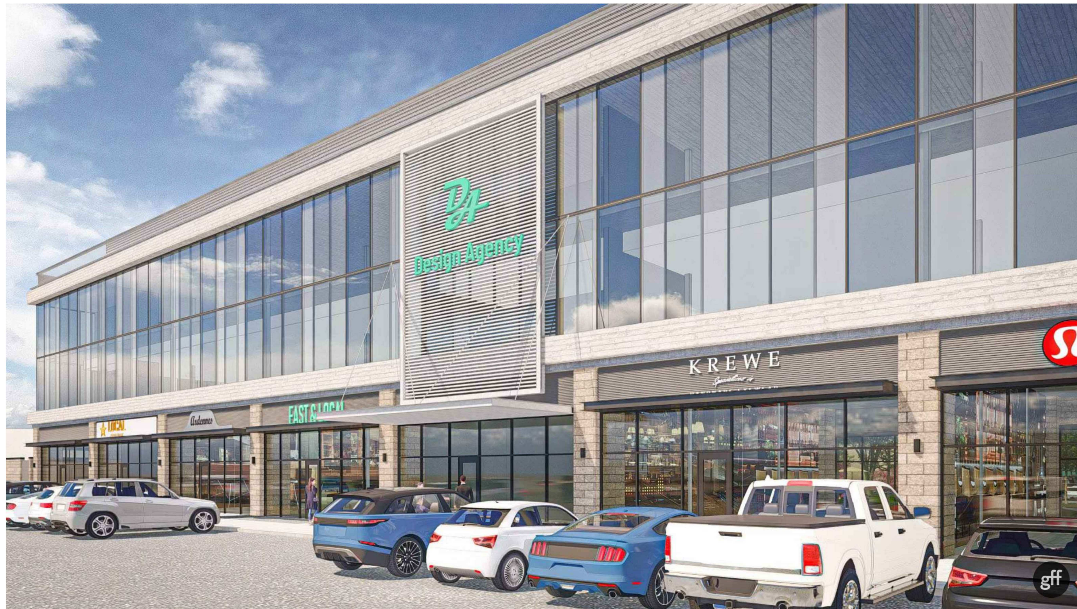
LOOKING SOUTHWEST AT OFFICE ENTRY
