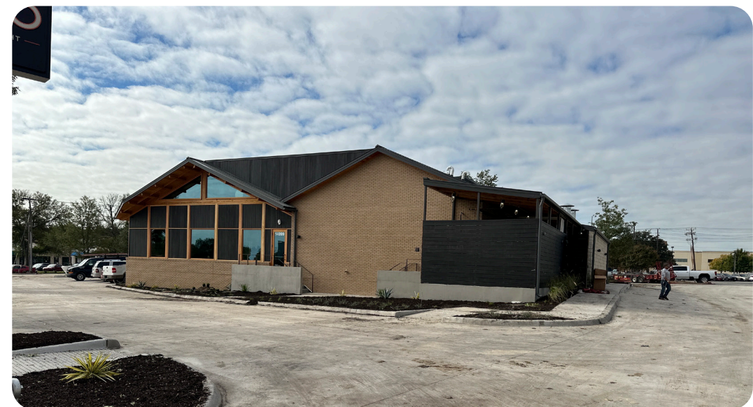
Building Photo - Proposed Mural Location Montfort Facade
