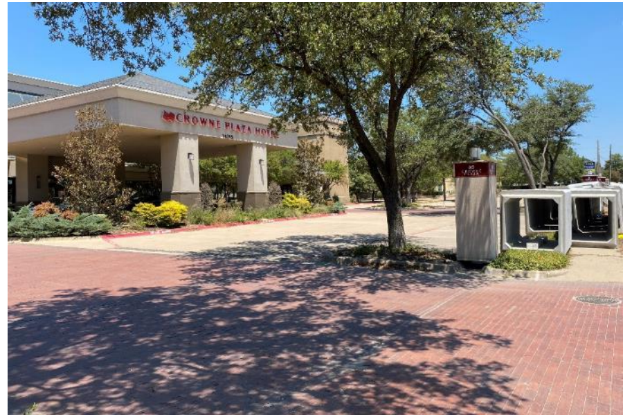
Existing Crowne Plaza Hotel
