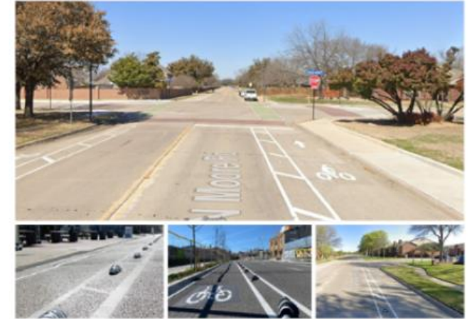
Example of Single Direction Buffered Bike Lanes
