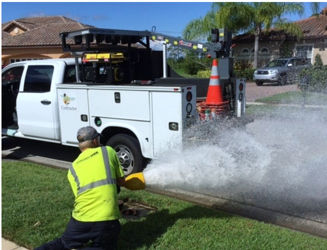
Hydrant Program in City of Cocoa
