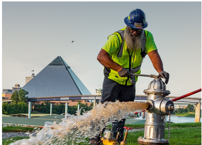
Hydrant Flushing in City of Memphis
