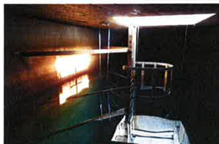
Interior Access Ladder
