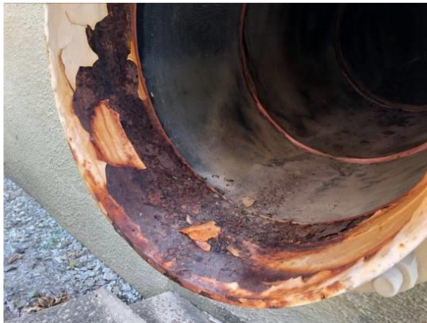
Photo No.31 – Overflow Pipe #2
