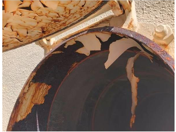
Photo No.30 – Overflow Pipe #1
