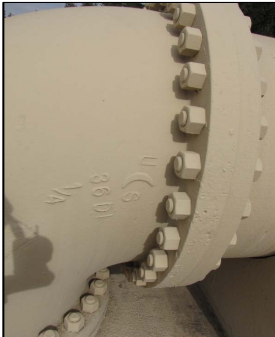
Photo 24 Inlet Pipe - 36 Inch Ductile Iron Class 53 Category: Operational
