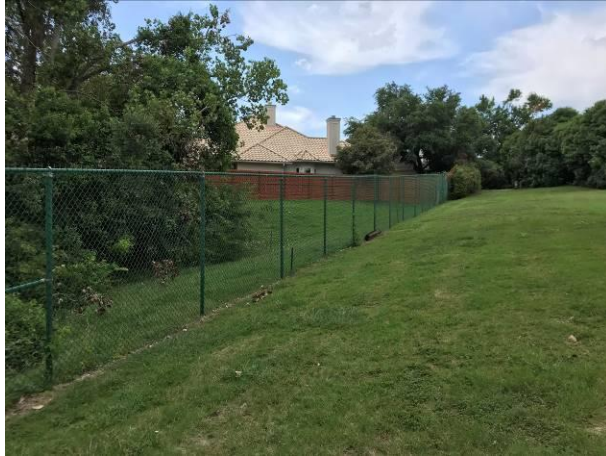
Photo No.23 – Chain Link Fence - West
