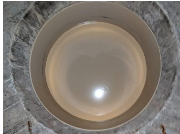
Photo No.40 Roof Vent Interior View
