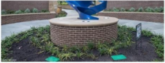
BASE: 2'x2' WITH BRICK AND CAST STONE FINISH TO MATCH BUILDING MATERIALS AND RECESSED UPLIGHTS
