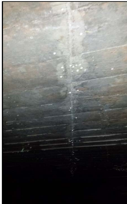
Photo 8 Interior Roof - Construction Joint Category: Structural
