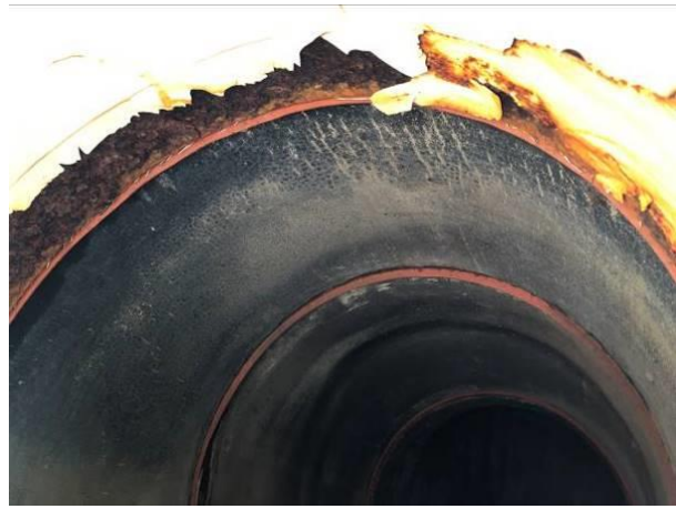
Photo No.32 – Overflow Pipe #2
