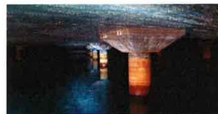
Interior Roof Structure and Columns
