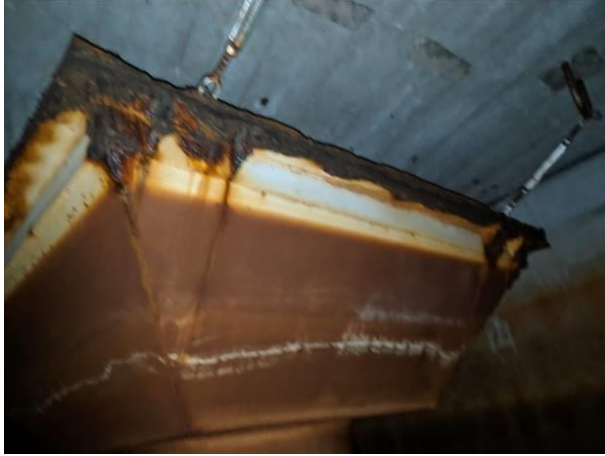
Photo No.33– Overflow Weir #1
