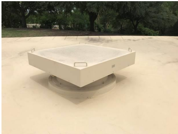
Photo No.39 – Roof Vent
