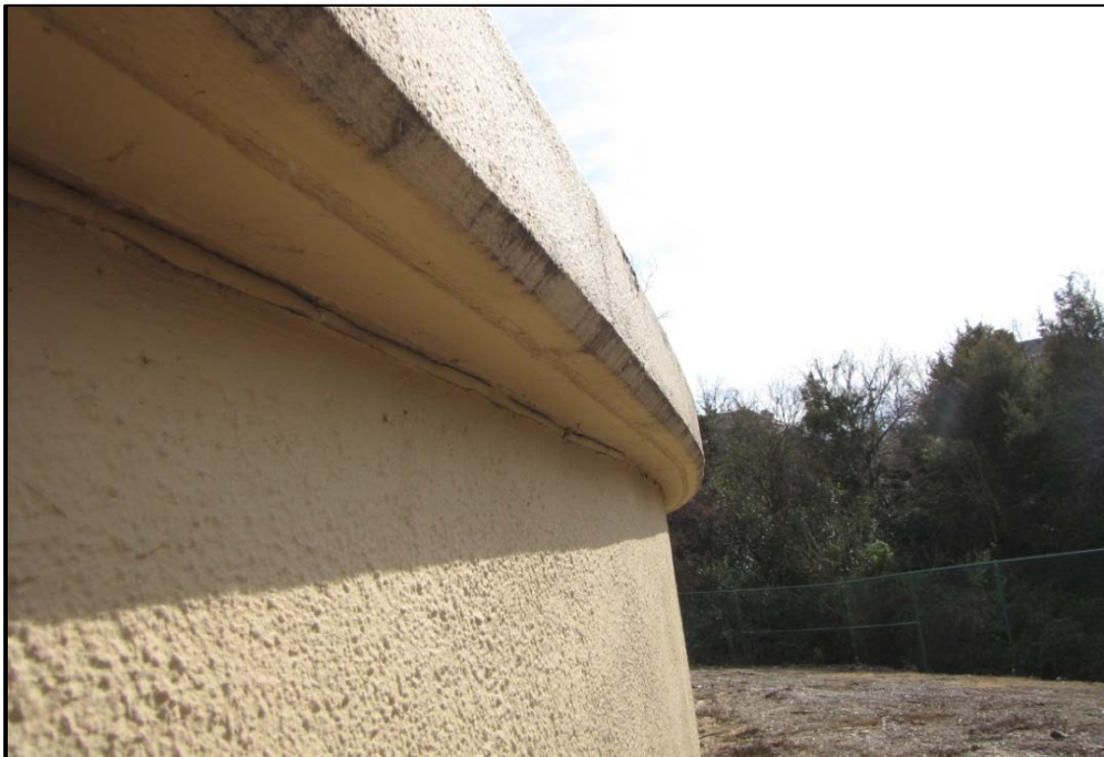
Photo 14 Shell Category: Structural
