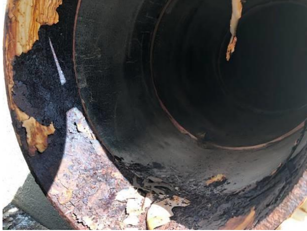
Photo No.29 – Overflow Pipe #1
