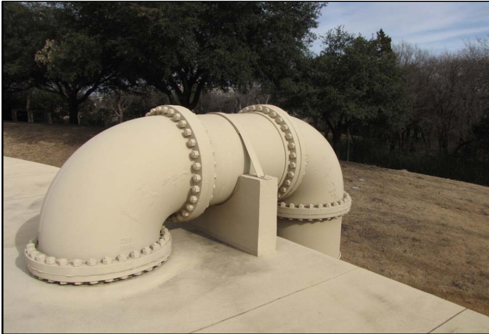
Photo 23 Inlet Pipe - 36-inch Ductile Iron Class 53 Category: Operational
