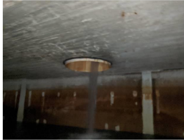
Photo No.28 – Inlet Pipe Interior
