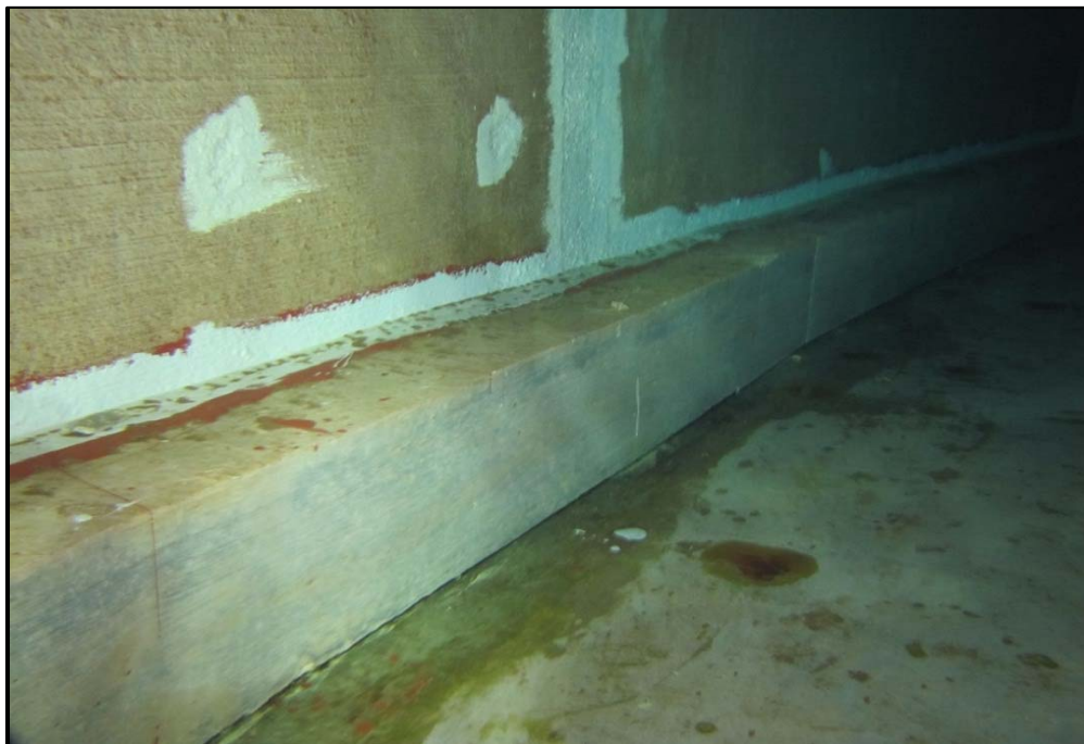
Photo 18 Water Stop Category: Structural
