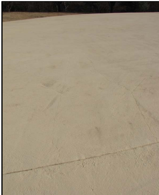
Photo 4 Roof - Construction Joint Category: Structural
