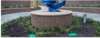
BASE: 2' 5x5' WITH BRICK AND CAST STONE FINISH TO MATCH BUILDING MATERIALS AND RECESSED UPLIGHTS
