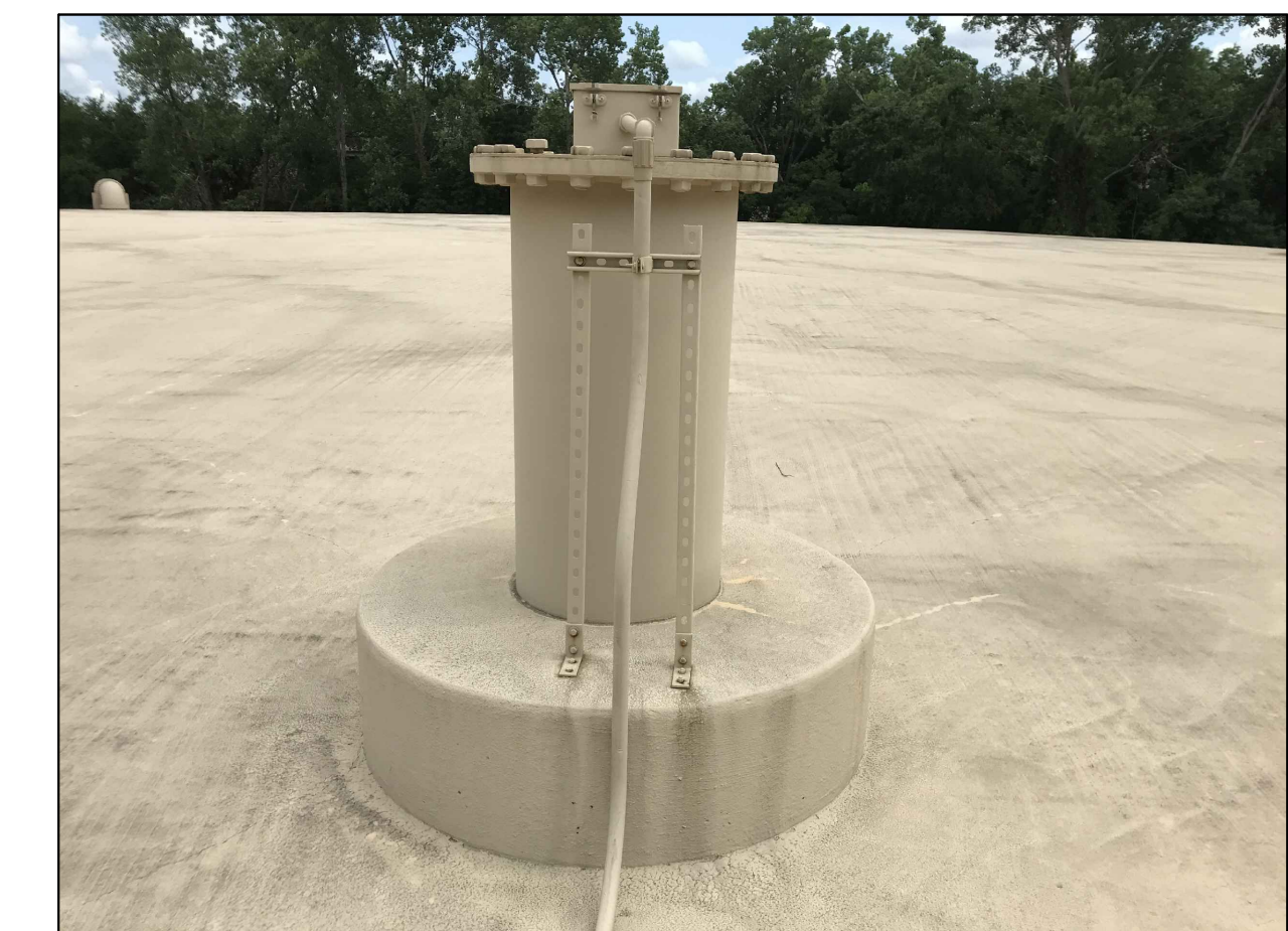
8 C11.0 EXISTING LEVEL INDICATOR REMOVE AND INSTALL NEW 24-INCH ROOF VENT ⚠️
