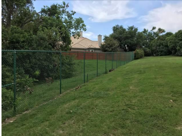
Photo No.23 – Chain Link Fence - West
