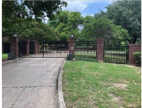
Photo No.22 – Northwest Gate
