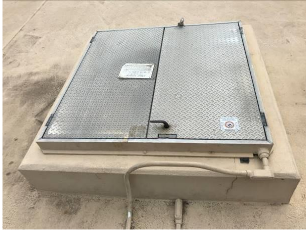
Photo No.19 – Roof Hatch
