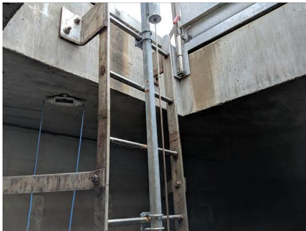
Photo No.17 - Interior Ladder
