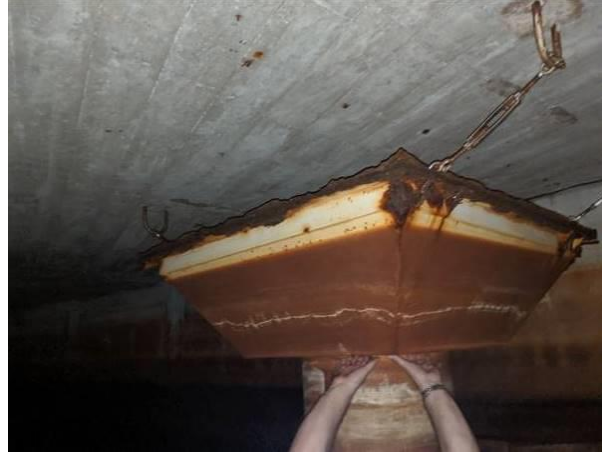
Photo No.34 – Overflow Weir #1
