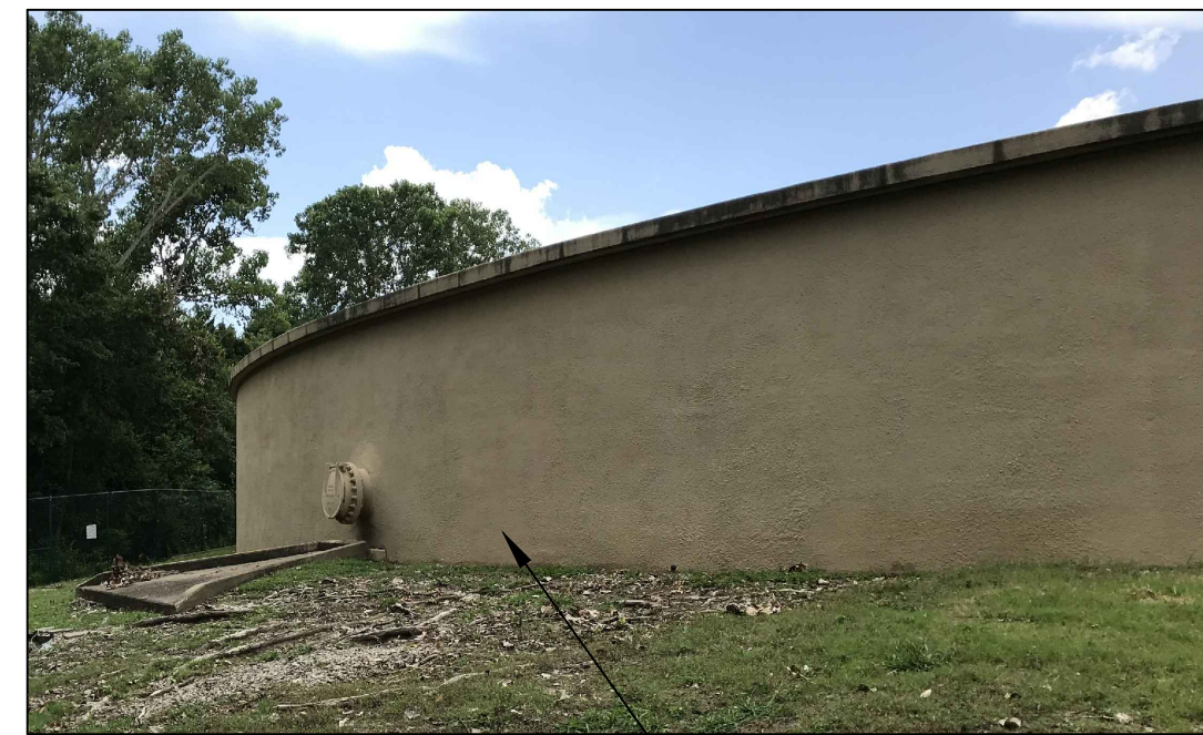
CONTRACTOR SHALL REPAIR EXISTING CRACKS AND COAT THE EXTERIOR SHELL PER CONTRACT DOCUMENTS
