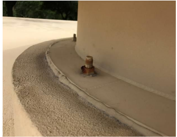
Photo No.46 – Carbon Coated Bolts (Exterior)
