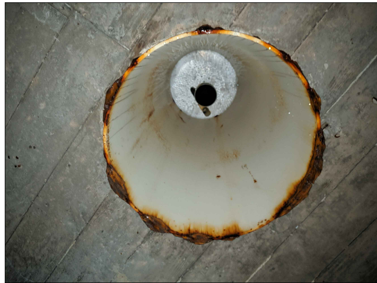
ROOF UNDERSIDE - INSTALL NEW ROOF VENT EXISTING LEVEL INDICATOR (5) S4.0 NO SCALE
