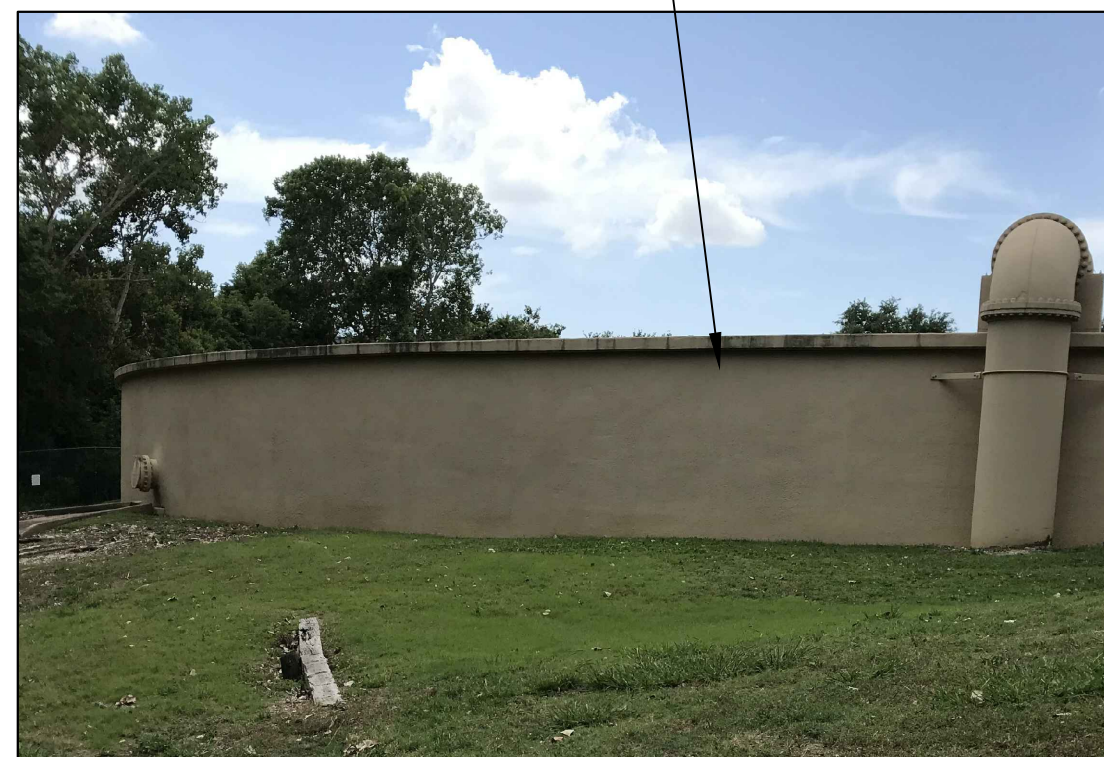
CONTRACTOR SHALL REPAIR EXISTING CRACKS AND COAT THE EXTERIOR SHELL PER CONTRACT DOCUMENTS
