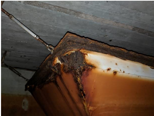
Photo No.35 – Overflow Weir #2
