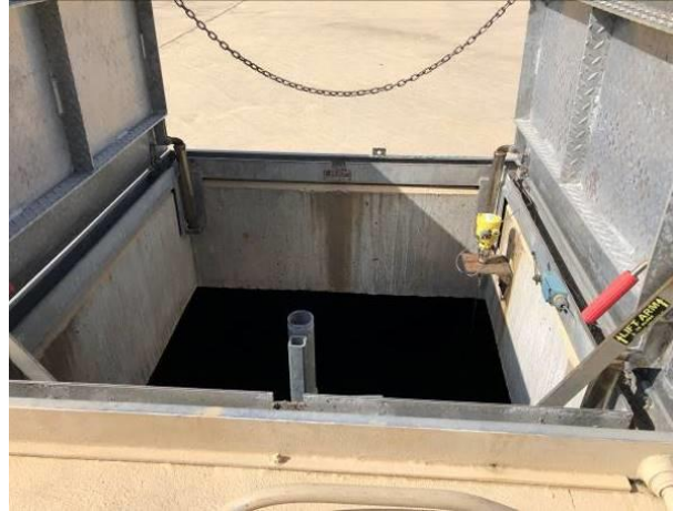
Photo No.20 – Roof Hatch
