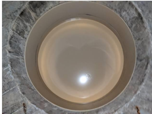
Photo No.40 Roof Vent Interior View
