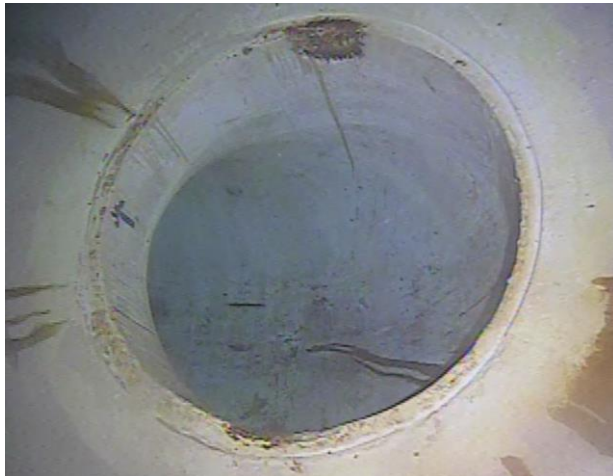
Photo No.29 – Outlet Pipe No.1
