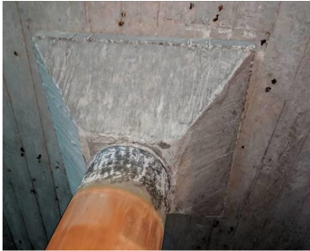
Photo No.11 – Existing Column
