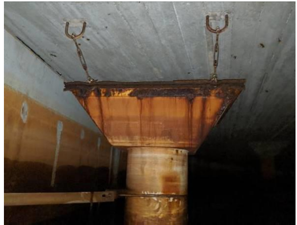
Photo No.36 - Overflow Weir #2
