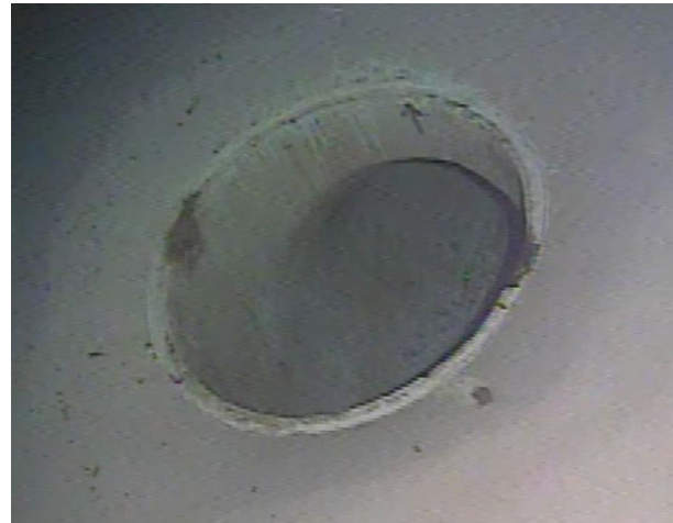
Photo No.30 – Outlet Pipe No.2
