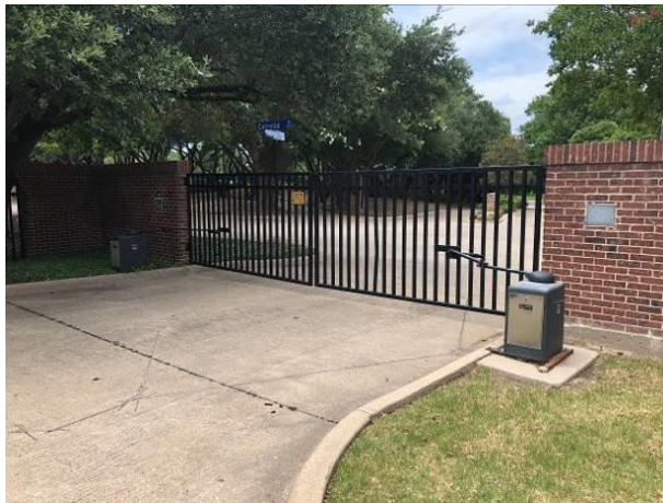
Photo No.211 – Northeast Gate
