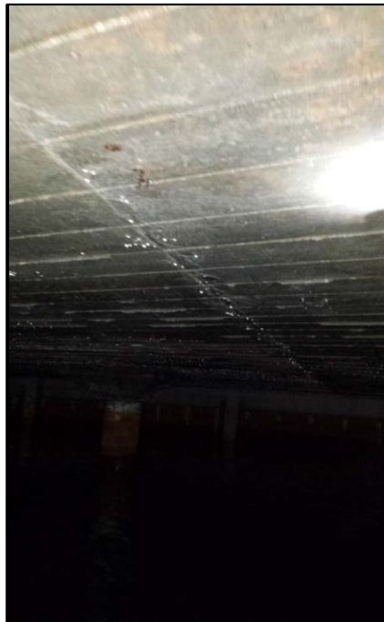
Photo 6 Interior Roof - Construction Joint Category: Structural
