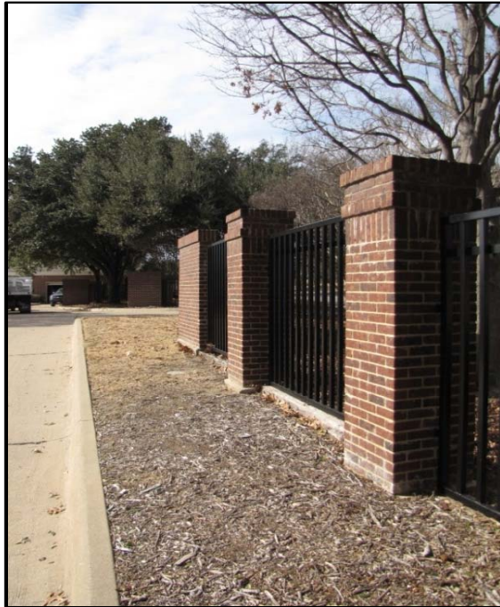
Photo 57 Perimeter Fence Category: Safety & Security
