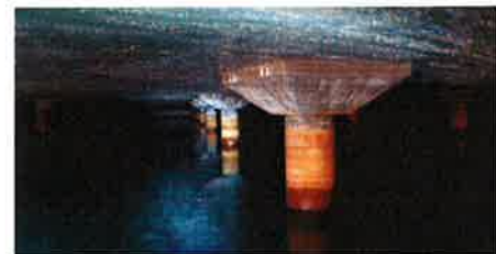
Interior Roof Structure and Columns
