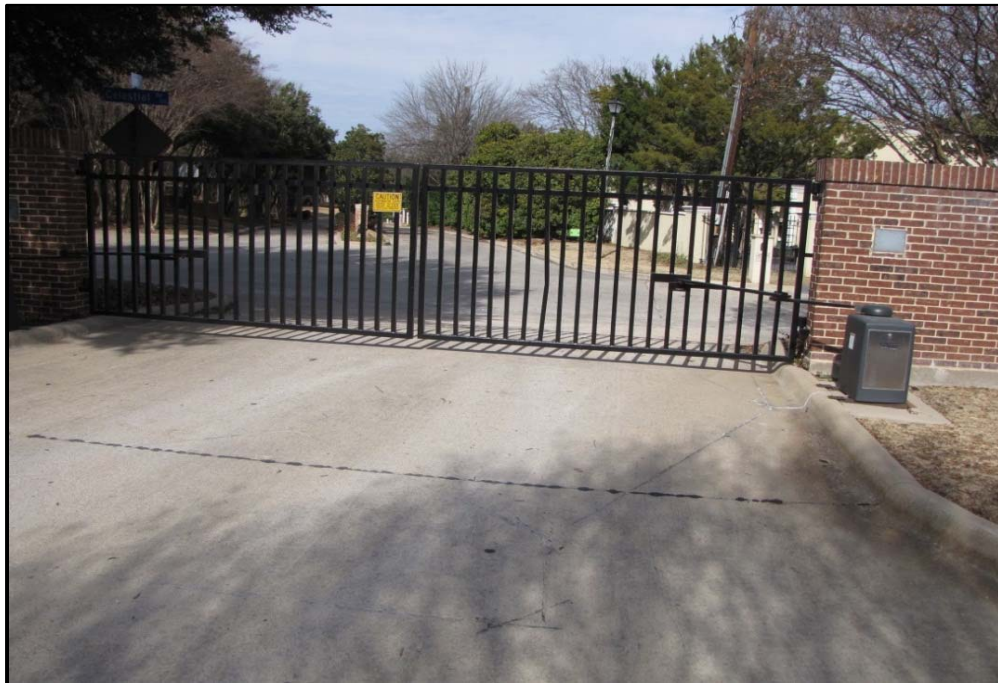
Photo 58 Gate Category: Safety & Security
