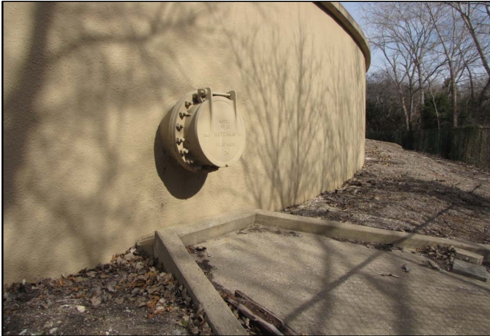
Photo 37 Overflow 2 - 24-inch Cast Iron with Concrete Splash Pad Category: Operational
