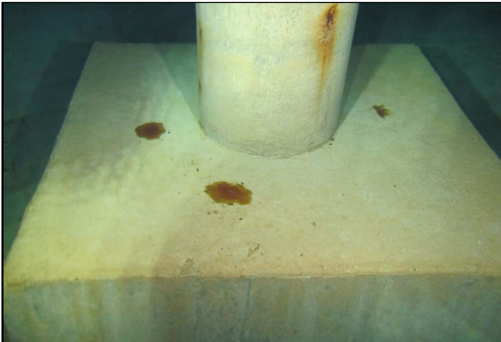
Photo 12 Column - 4-foot Square Base with 16-inch Column Category: Structural
