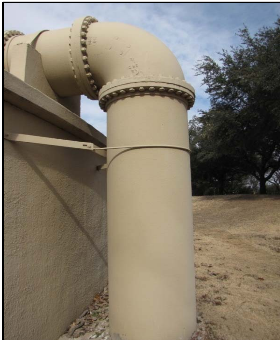
Photo 22 Inlet Pipe - 36-inch Ductile Iron Class 53 Category: Operational
