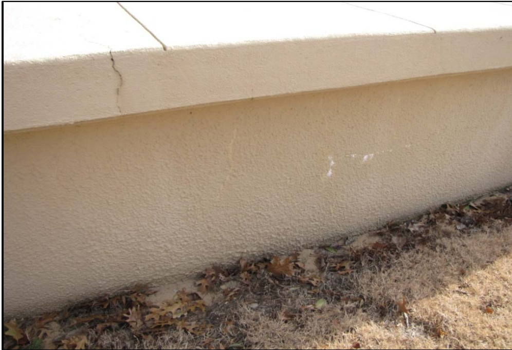
Photo 3 Roof Category: Structural
