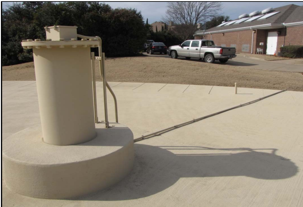
Photo 46 Pipe - 24-inch Steel Pipe for Sonic Level Transmitter (Abandoned) Category: Operational
