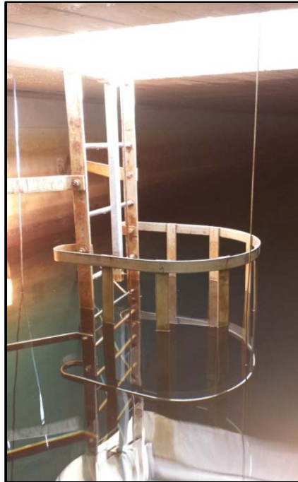
Photo 53 Interior Ladder - Stainless Steel Ladder Cage Category: Safety & Security
