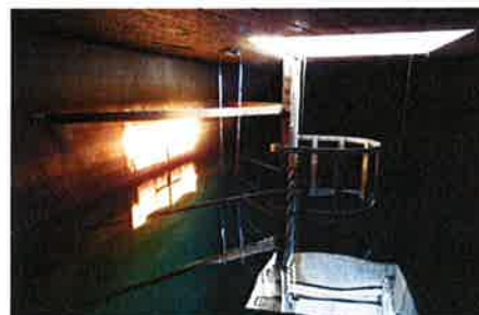
Interior Access Ladder
