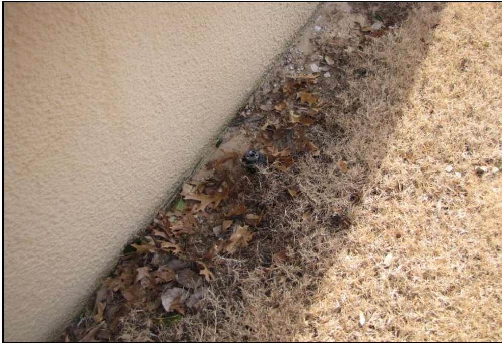
Photo 15 Shell with Sprinkler Head Category: Structural
