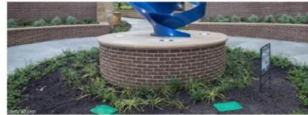
BASE: 2 5'x5' WITH BRICK AND CAST STONE FINISH TO MATCH BUILDING MATERIALS AND RECESSED UPLIGHTS
