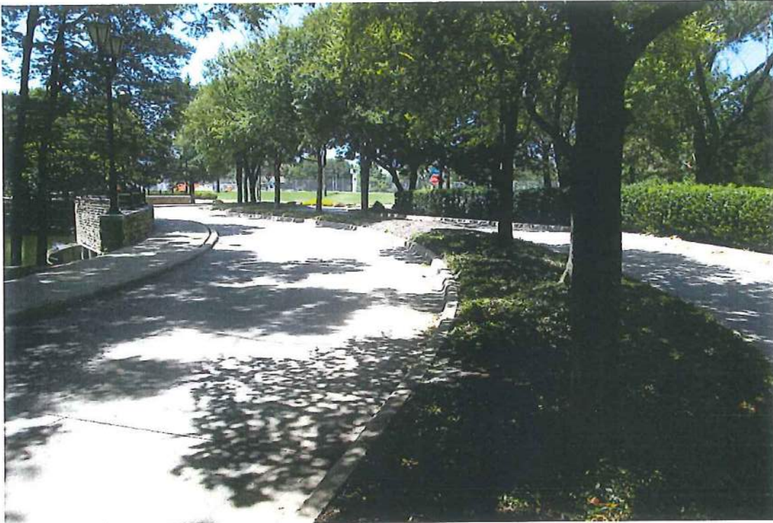
BRIDGE ROADWAY LOOKING NORTH
