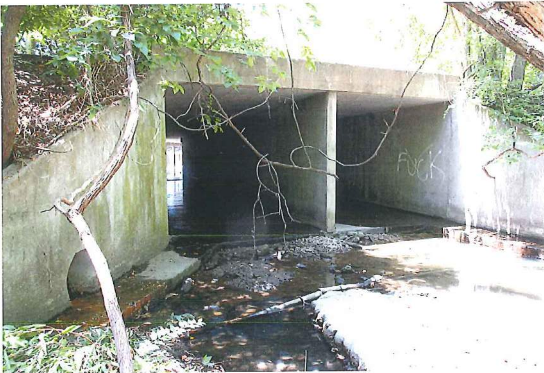
BRIDGE ELEVATION LOOKING NORTHWEST
