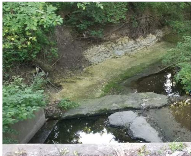
Photo 4: Downstream Looking East
