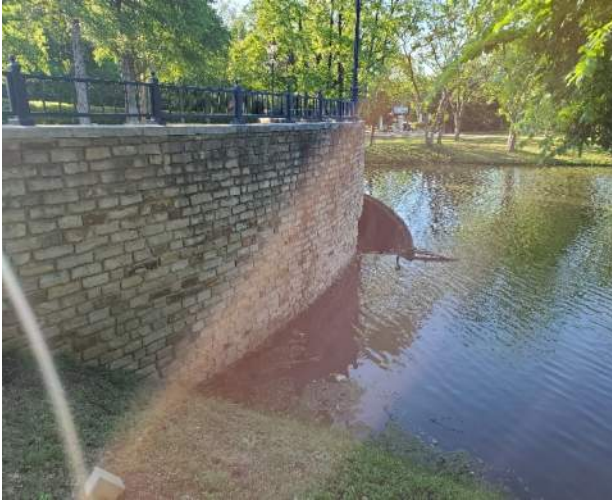
Photo 9: Upstream Channel Banks (North)
