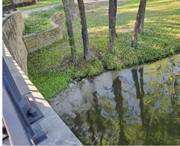
Photo 10: Upstream Channel Banks (South)
