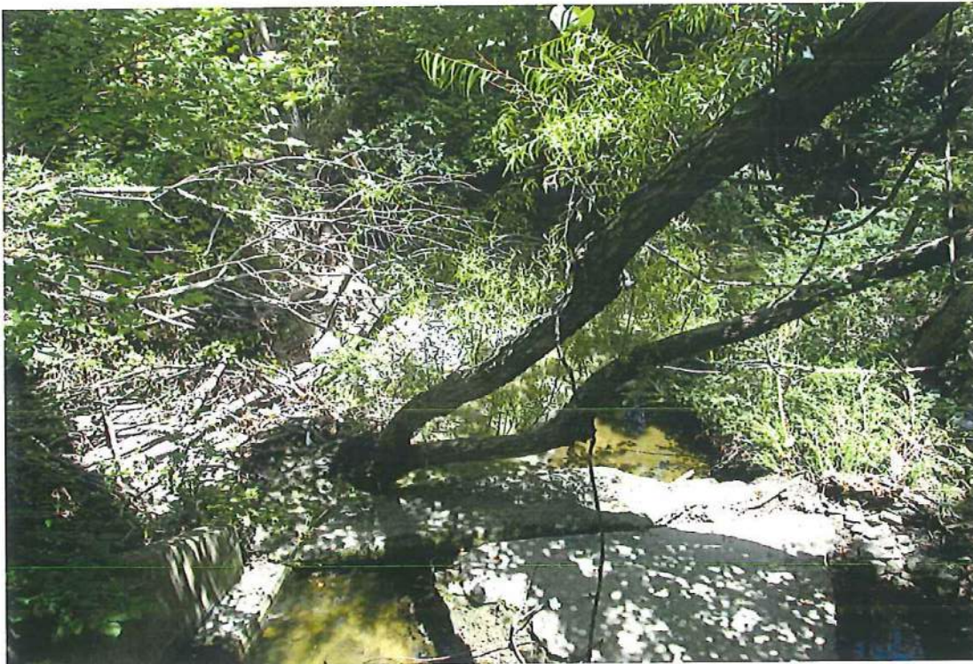
DOWNSTREAM VIEW FROM BRIDGE LOOKING EAST
