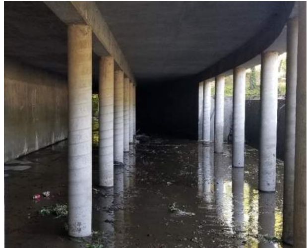
Photo 20: Culvert Columns at Spillway
