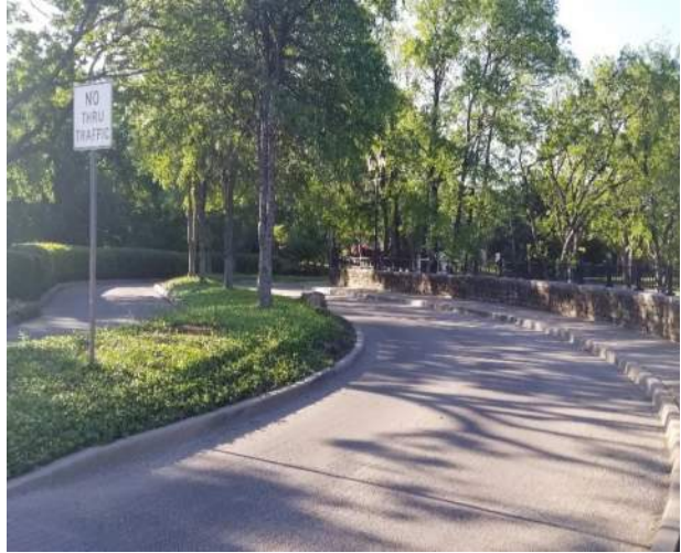
Photo 6: Roadway Looking South
