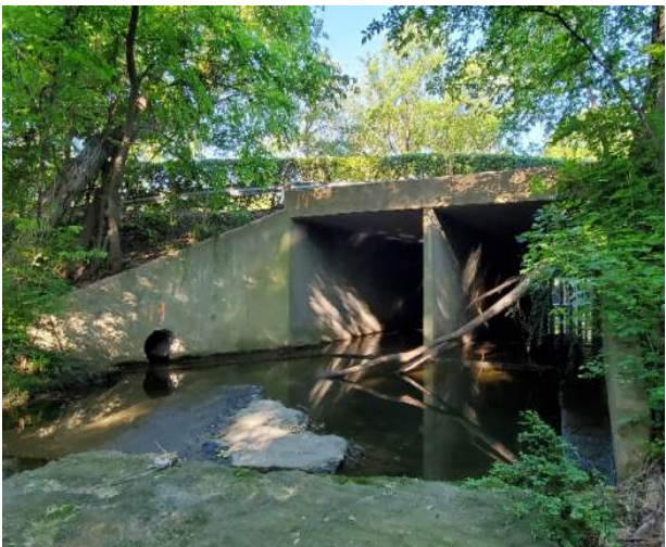
Photo 3: Downstream Looking West
