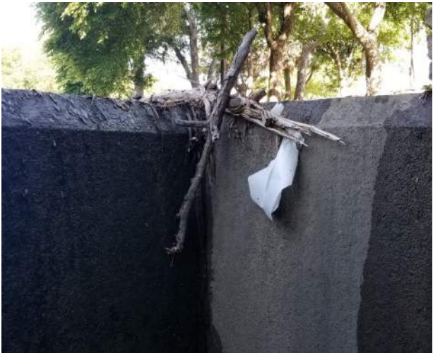
Photo 15: Spillway Debris
