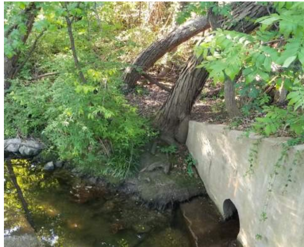
Photo 12: Downstream Channel Banks (South)
