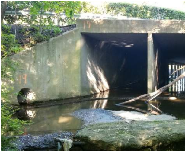
Photo 19: Wingwall and Headwall
