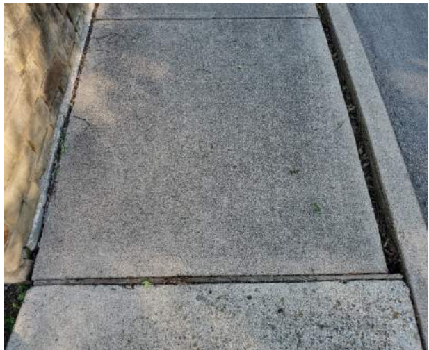
Photo 8: Sidewalk Joint
