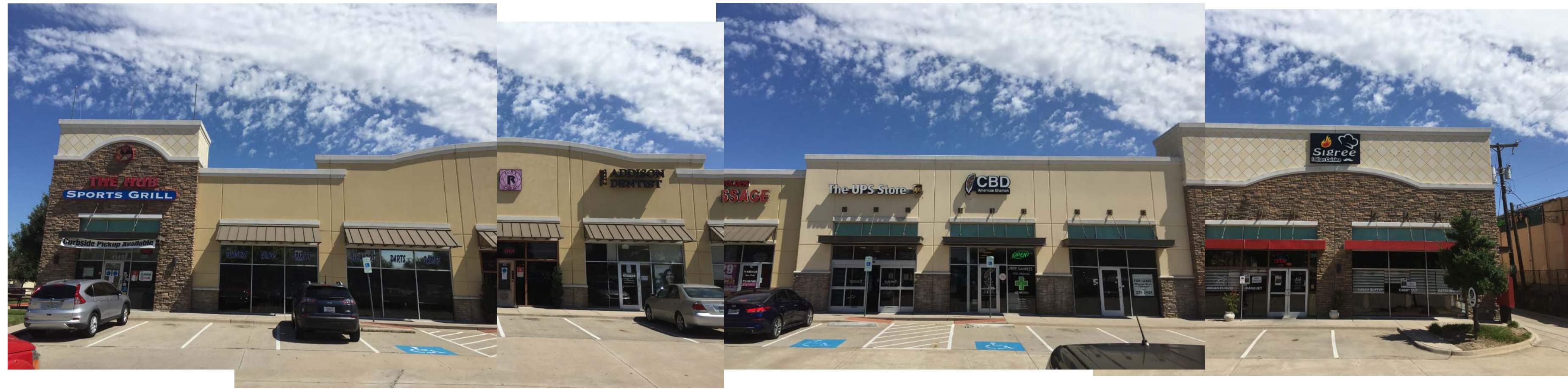
A EXISTING SOUTH FACADE: 4145 BELT LINE Scale: NONE
