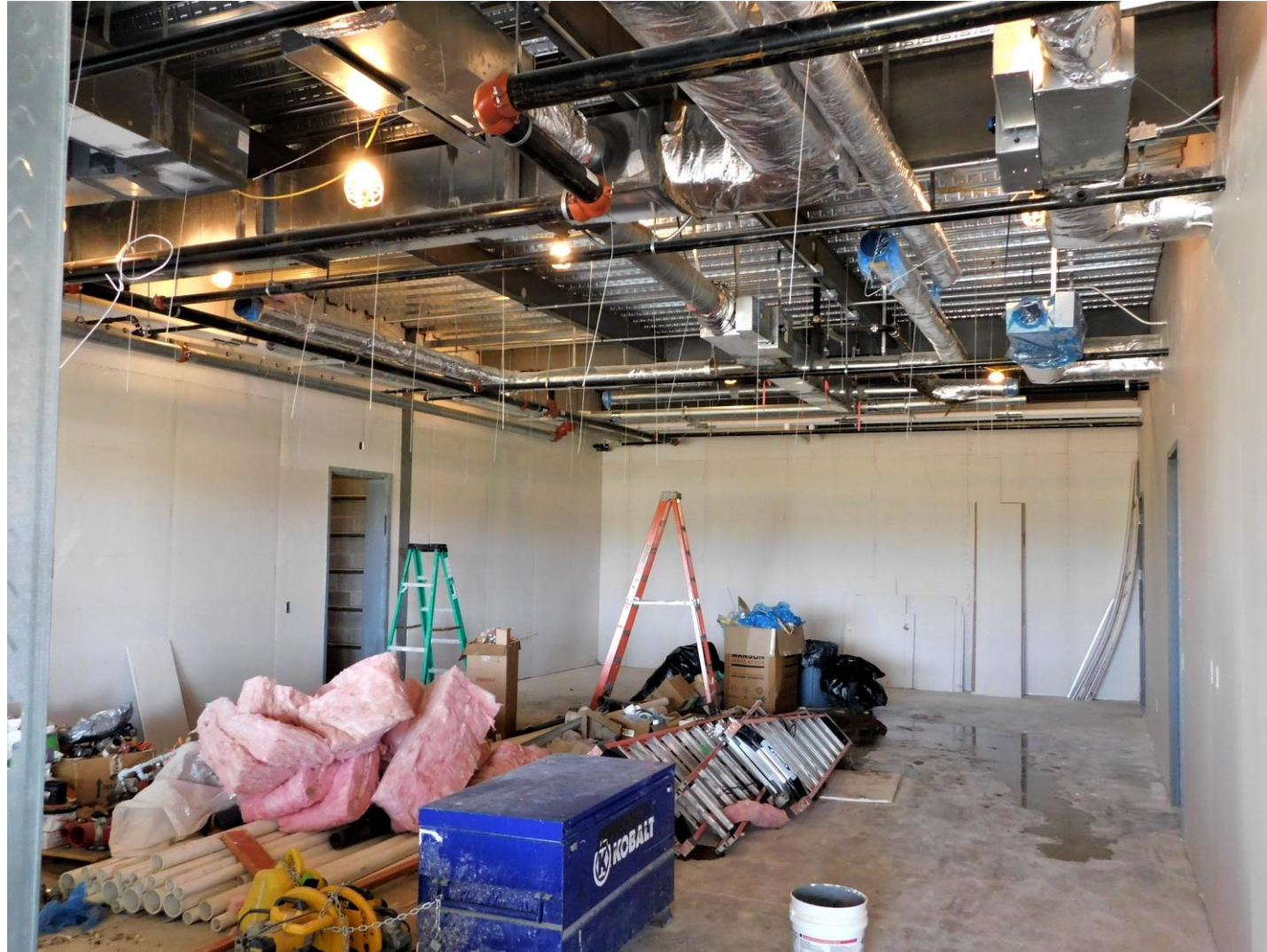
First floor processing area (September 25, 2020).
