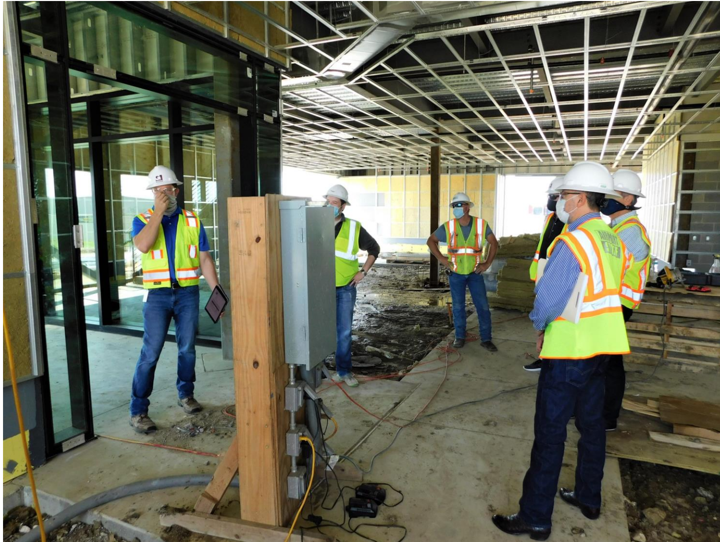
The breezeway area where landscaping changes will be made (September 25, 2020).
