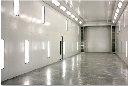
CWD On-site Container Paint Facility
