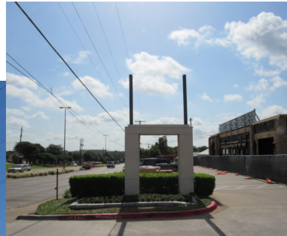
CURRENT STATUS OF D/F PYLON SIGN - EXISTING I-BEAM STEEL SUPPORTS TO BE RE-USED w/ NEW SIGN CABINET
