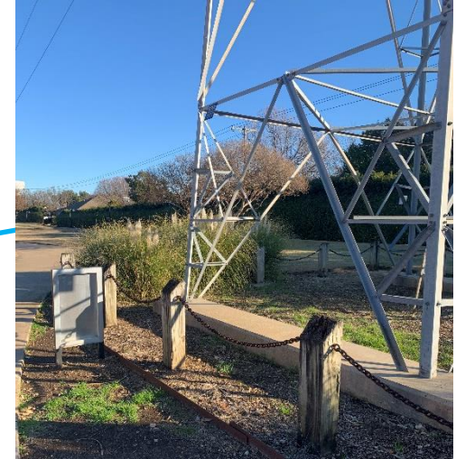
Structure Zone - Requires a 25 Foot perimeter from tower base. Turf Planting Only.
