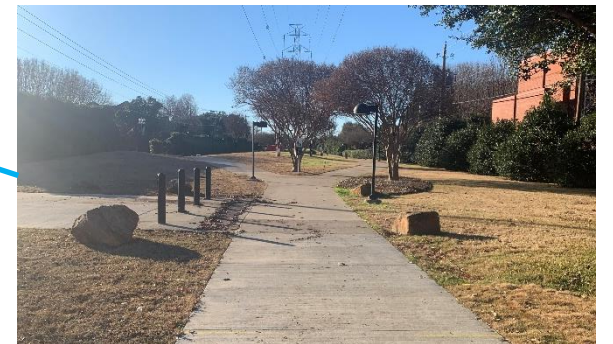
Temporary removal boulders, bollards, lights and permanent removal of trees in construction path.
