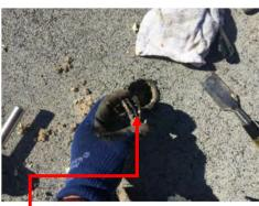
Roof membrane weak and delaminated
