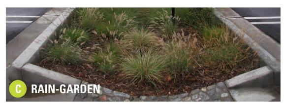
Description - Catch and filter stormwater runoff from the streets by converting concrete flumes into rain-gardens. Cost - \$43,500
