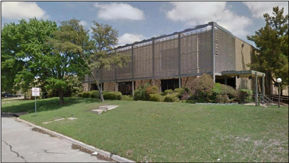
Office/light industrial building on Beltwood
