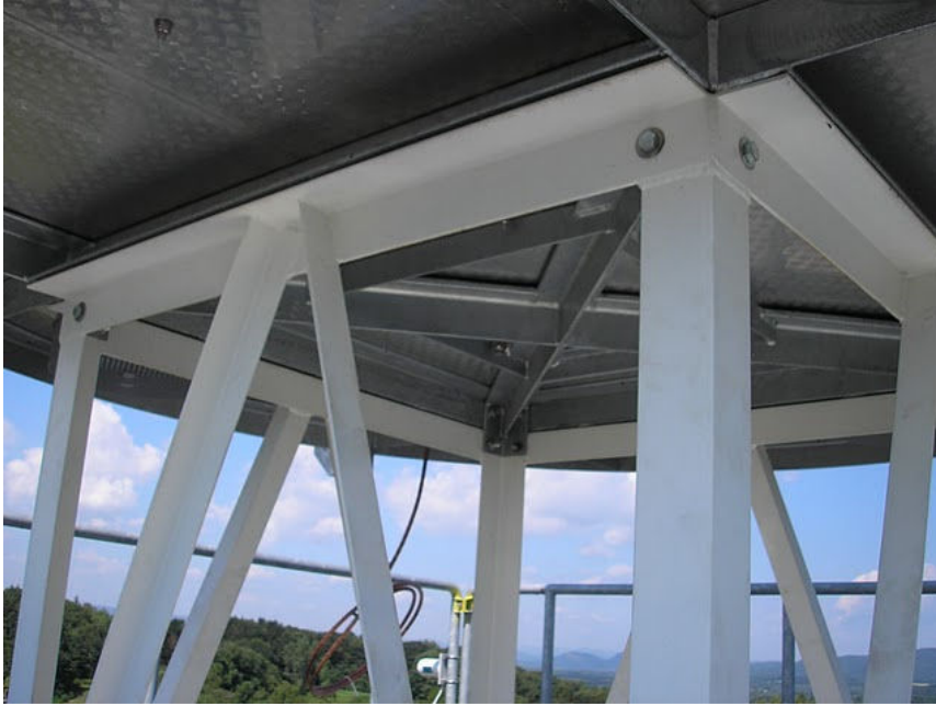
Figure 20 - Radar mount elevated off the platform
