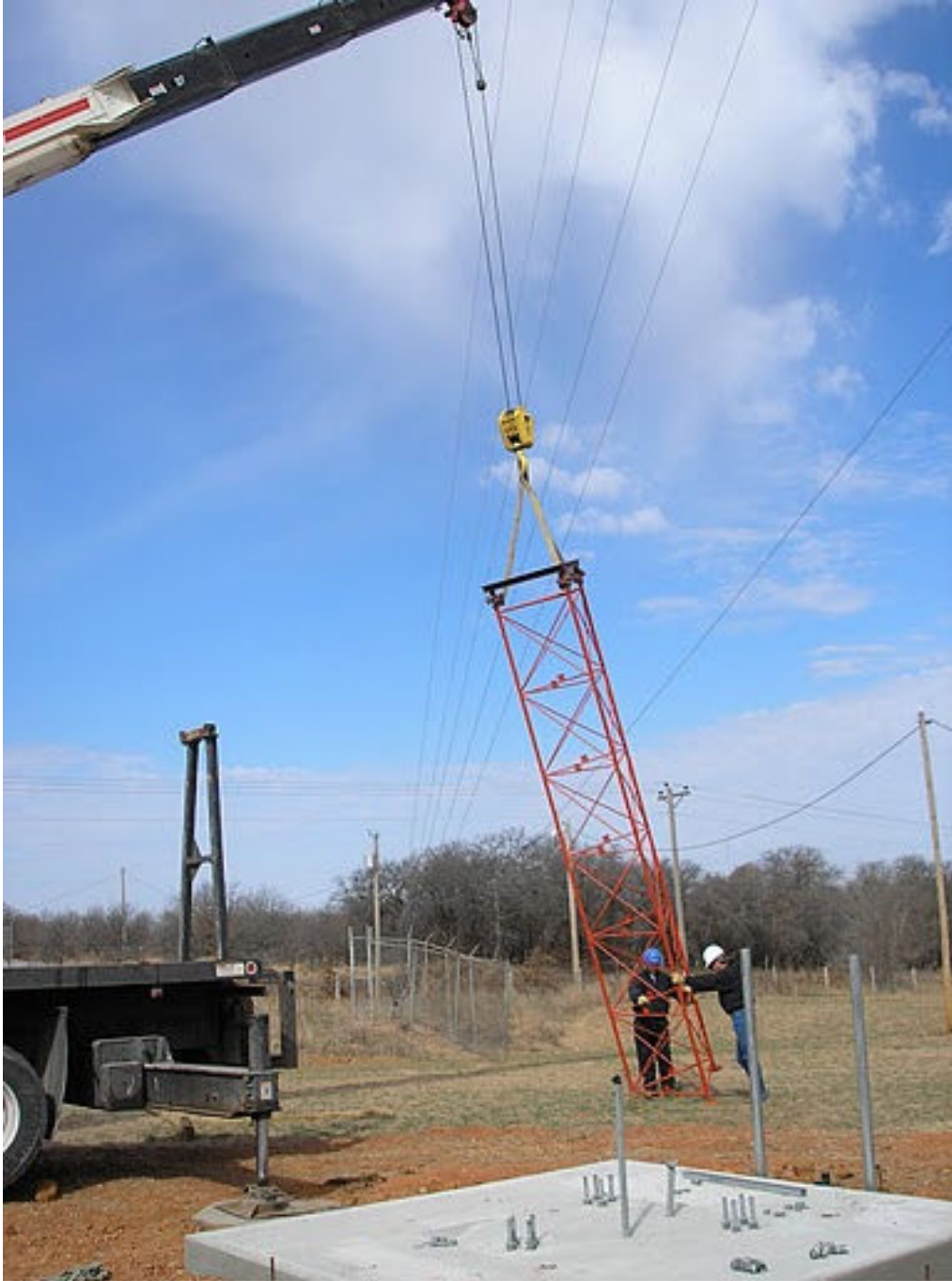
Figure 4 - Tower lifted into place
