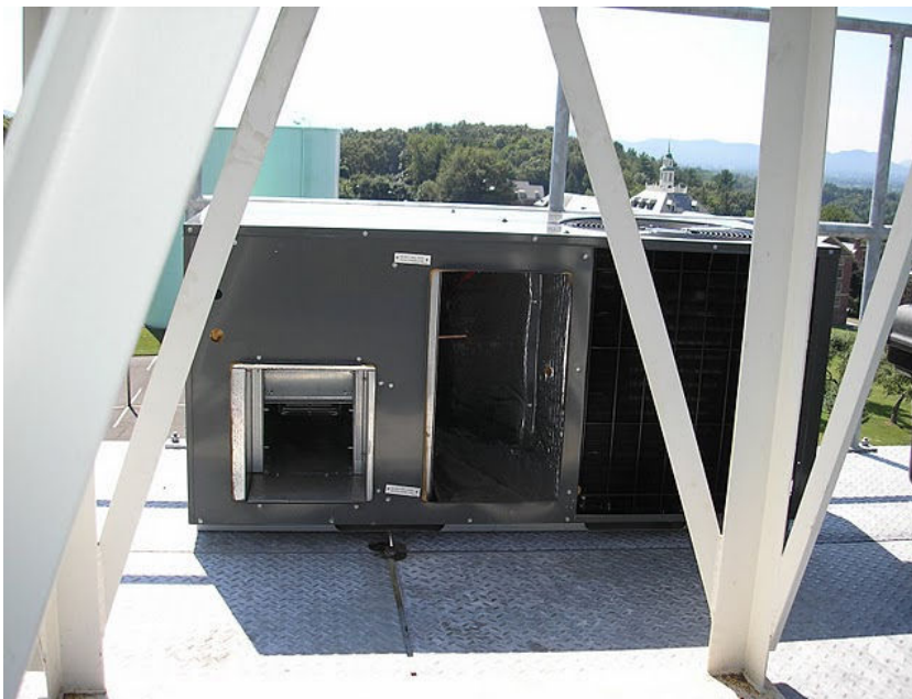
Figure 21 - HVAC unit craned up to tower top platform
