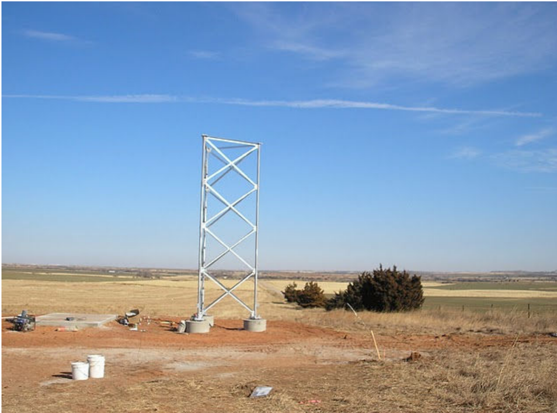
Figure 12 - Ground preparation for Tall Tower Installation
