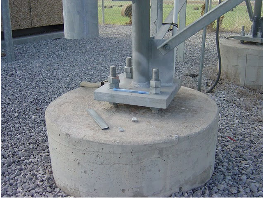
Figure 13 - Tower feet anchored to reinforced concrete cylinders.
