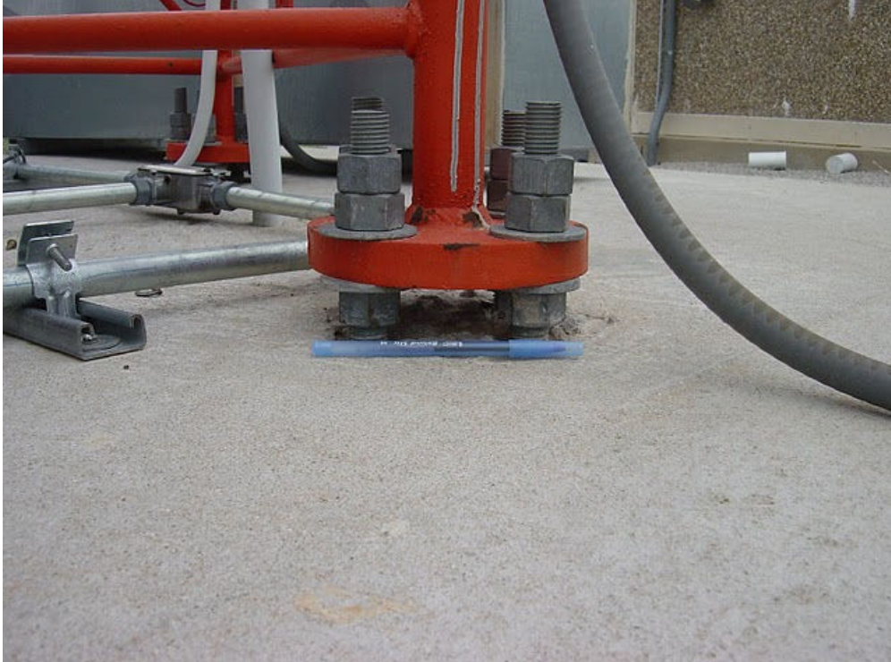
Figure 5 - Side view tower anchoring and conduit
