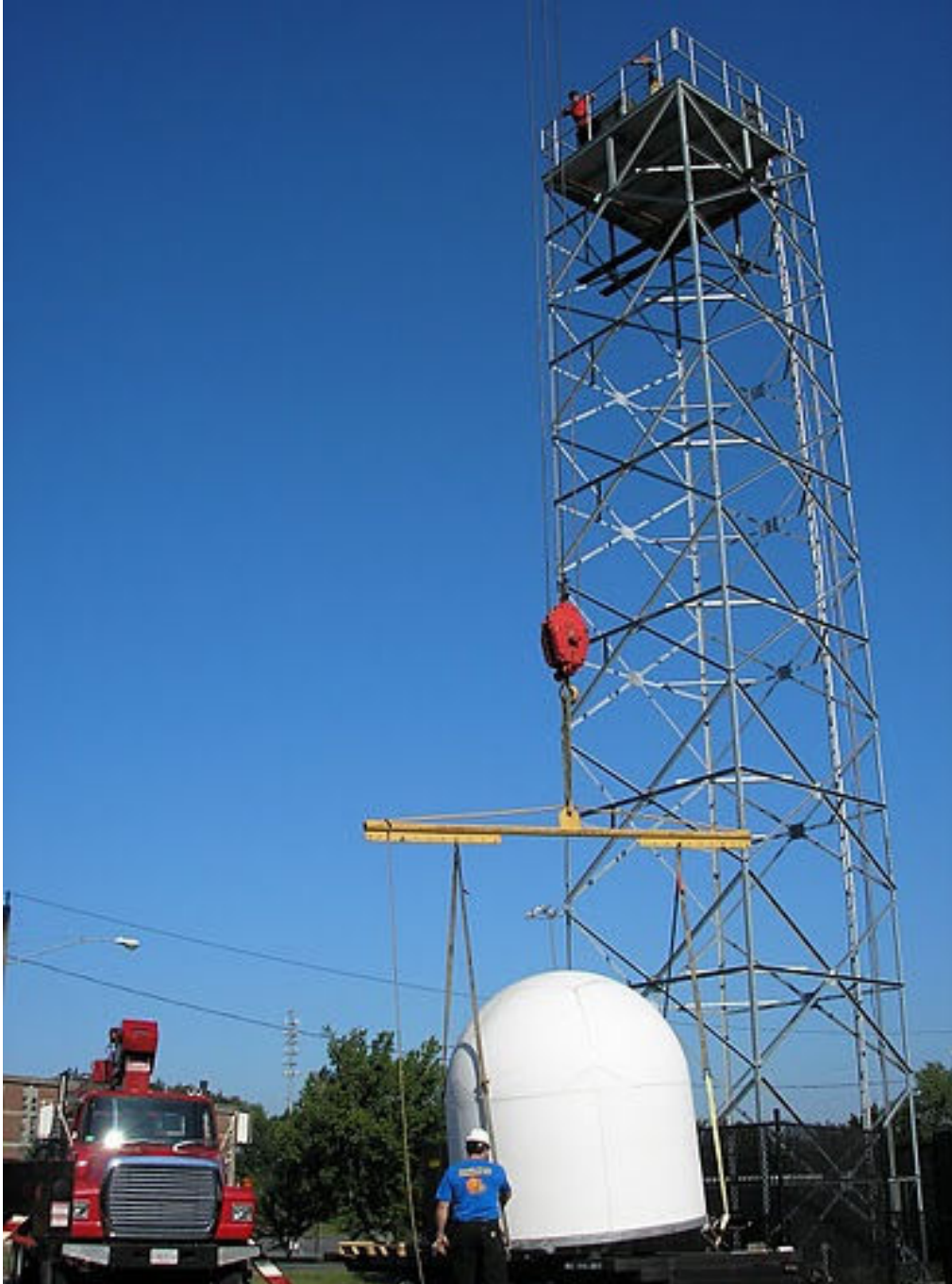
Figure 19 - Radar is craned onto a platform constructed at the top of the square tower
