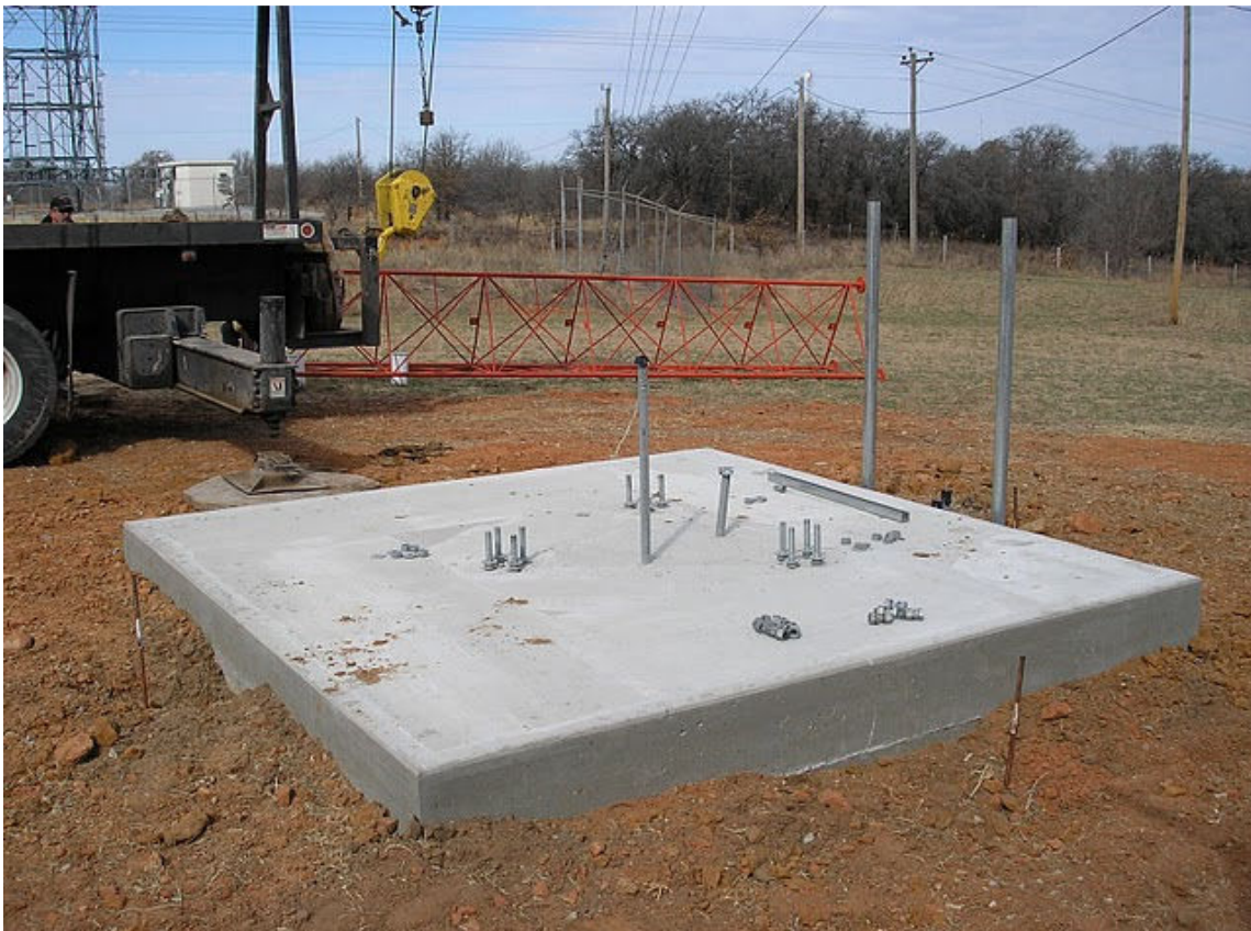
Figure 3 - Poured foundation, anchor bolts, trenched-in conduit
