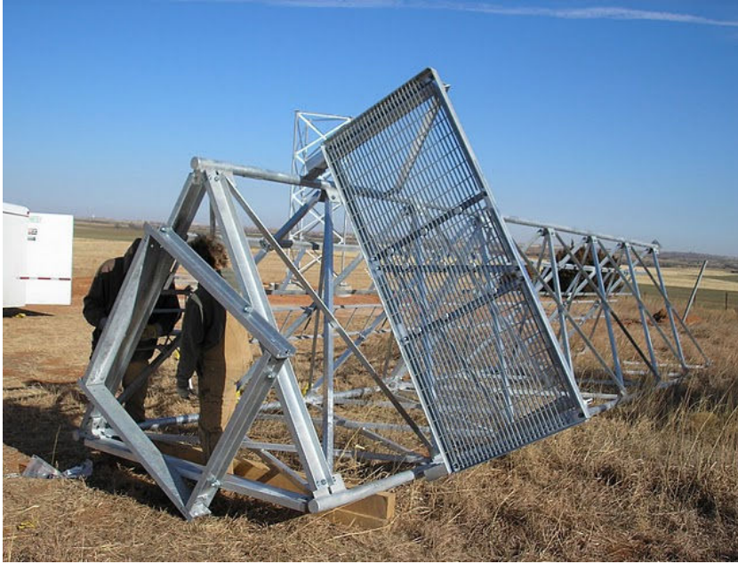
Figure 15 - Tower top with small platform
