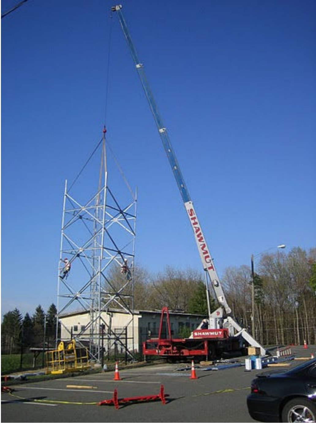
Figure 18 - A square tower is craned into place
