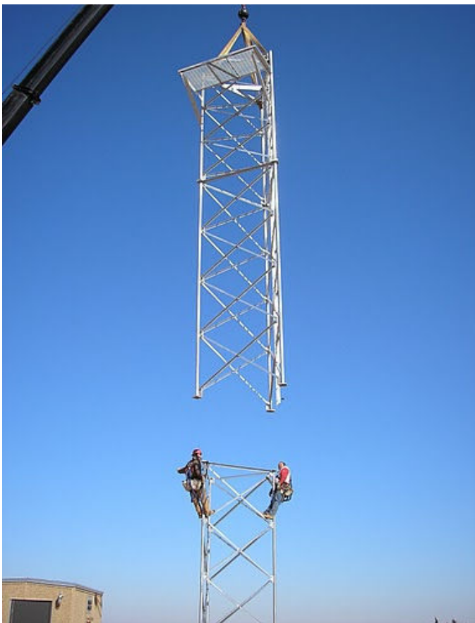
Figure 16 - Tower top craned into place
