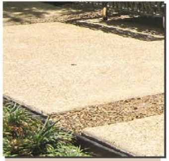
INTEGRAL COLORED CONCRETE 2
