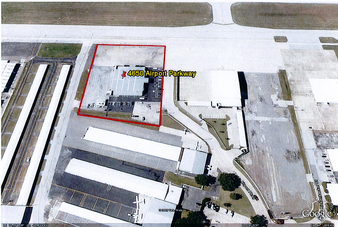
View of 4650 Airport Parkway facing west with the Pepsico Hangar to the right.
