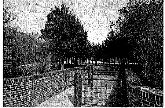
Addison TXU Right-of-Way
